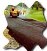
Asphalt (road paving) materials are heated up (making them less viscous) so they can be poured easily before it hardens.
